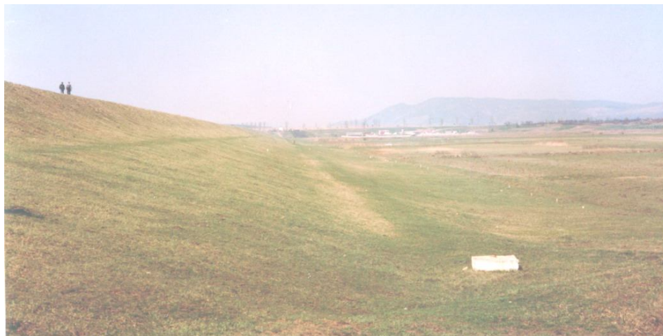
Fig. 2. – The downstream facing of the dam
