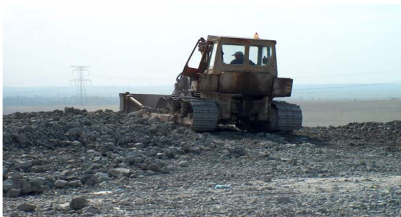
Fig. 3. The compaction and leveling of the industrial wastes storage face.
