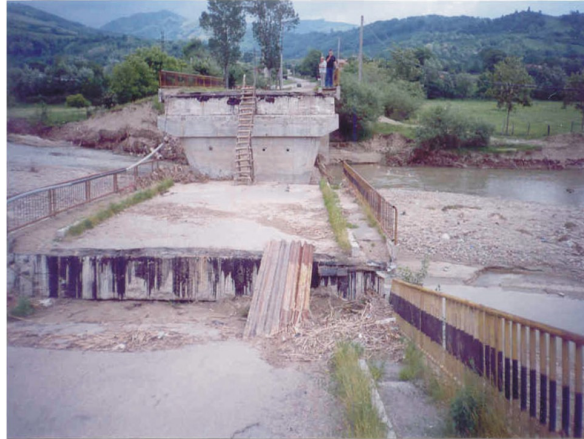
Fig. 3 – Bridge between Bâscenii de Sus and Zeletin destroyed by the high-water of May 2005.
