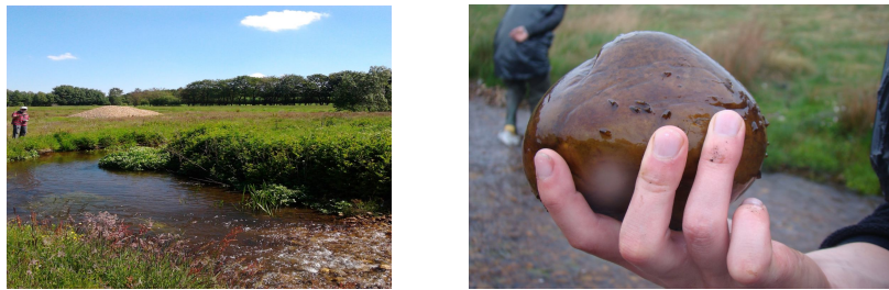
Fig. 8 – The use of river stone to stabilize the new stream thalweg of the remeandred Odderbae River in Denmark; development of fauna and flora (authors photo).
