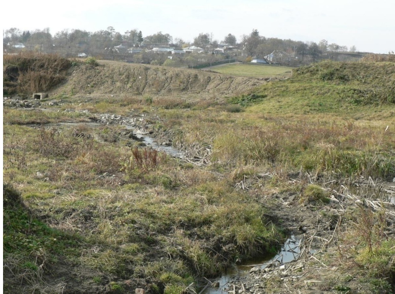
Fig. 2 – Downstream view of the embankment and the partially stoppered breach.
