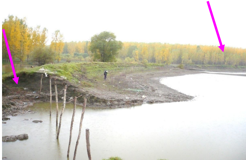
Fig. 8 – Breaches in the contour dyke.
