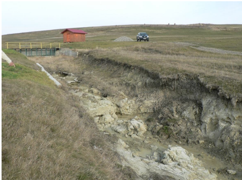
Fig. 7 – Spillway fast channel – ravine.
