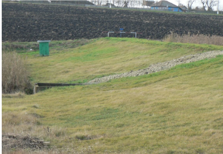
Fig. 6 – Downstream slope of the embankment—eroded area.
