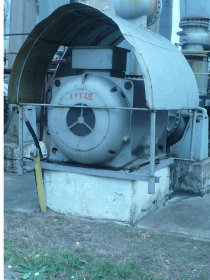
Fig. 9 The electrical pump EPT 2/II within CET South Timișoara.
