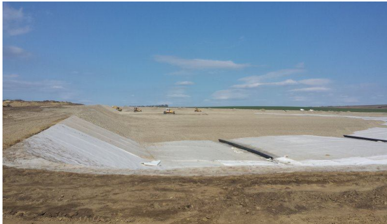
Fig. 7– Mounting the leachate drainage layer.
