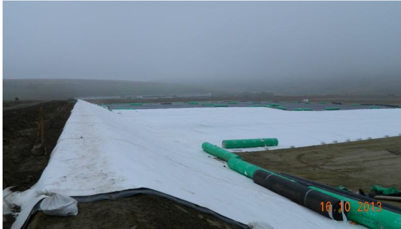
Fig. 6 – Mounting the geotextile.
