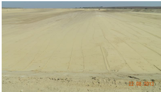
Fig. 4 – The sealing mineral layer.
