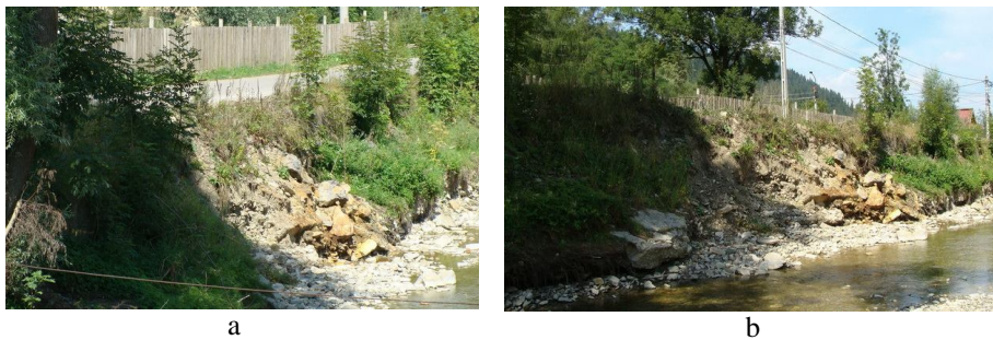
Fig. 7 – Details on the erosion phenomenon of Voroneț River bank and the degradation of DJ 177D in Voroneț District; a – blocking of the shore erosion with large stones; b – highlight of the erosion area on the shore protection line (Luca, 2016).
