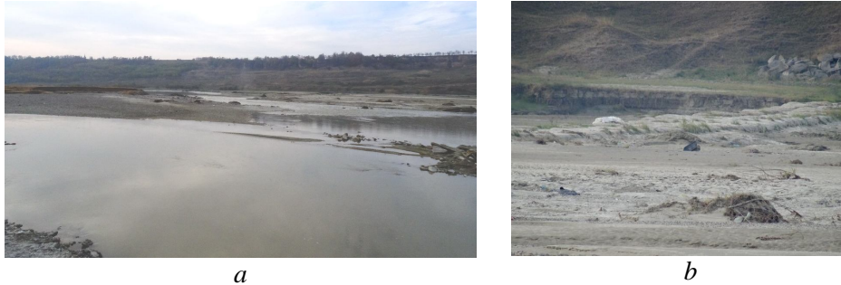
Fig. 7 – The state of the riverbeds separation area around the catchment: a – general view of the separation area with closing dyke; b – detail on the dyke degradation, year 2018 (Photo author).
