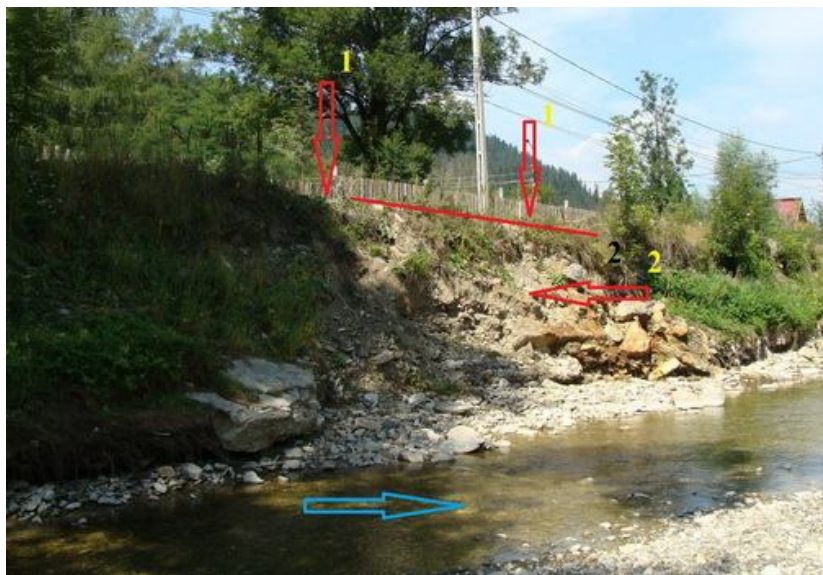
Fig. 5 – General view of the DJ 177D degradation located in Voroneț District due to the erosive action of the water during floods: 1 – the erosion of the road shoulder with ingress in the road; 2 – the shore protection fully degraded and shore erosion (Photo Luca, 2016).
