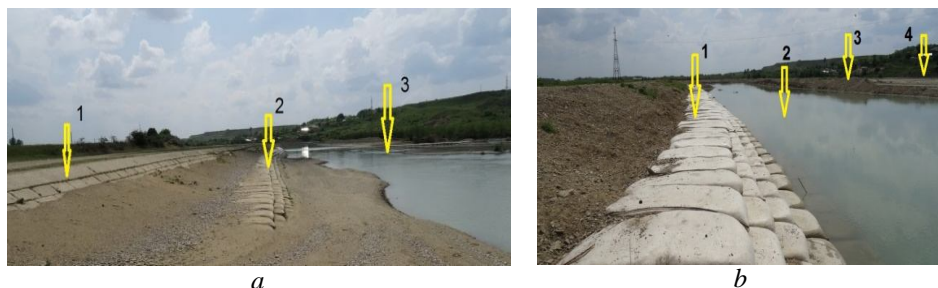
Fig. 5 – General view left bank shore protection downstream of deviation area: a – left bank with the old and new left bank shore, 1 – concrete slabs, 2 – geocontainers, 3 – deviated riverbed; b – geocontainers shore protection, year 2015 (Photo Luca, 2015).
