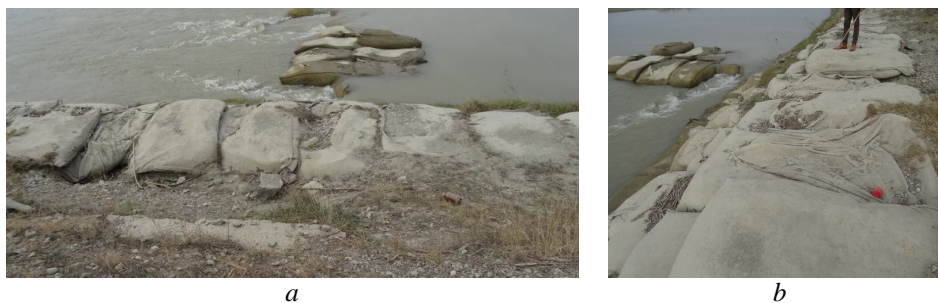
Fig. 9 – Degradation of shore protection made of geocontainers on the deviated minor riverbed, year 2018; a – elements degraded by floaters in water; b –geocontainers degradation on the superior side of the shore protection (Photo Luca, 2018).
