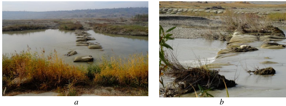
Fig. 8 – Aspects regarding the degradation of bottom sills on the deviated minor riverbed, year 2018; a – general view; b – detail on the bottom sill state (Photo Luca, 2018).
